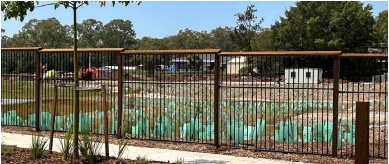
Plate 7: Koala exclusion fencing similar to that proposed
