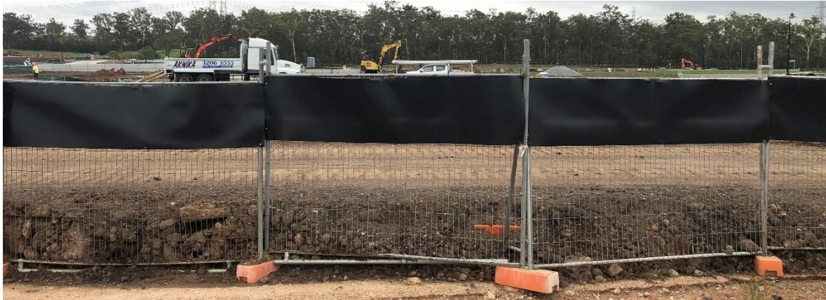
Plate 8: Temporary fauna exclusion fencing installed on an active construction Site
