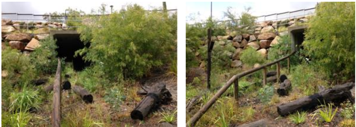
Inset 12: Indicative example of a fauna underpass with fauna furniture (note the Proponent's proposal will attach the poles to the wall of the culvert and will use a much smaller concrete apron to allow more planting around the portal). Further, rocks will be provided within the culvert to provide cover for small terrestrial species.
