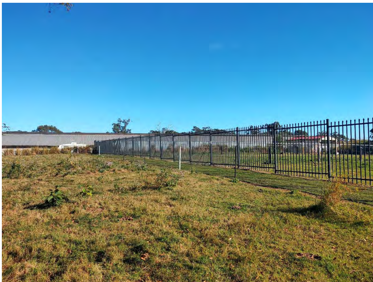
Plate 10 – Exclusion fence on the southern boundary of Lot 3 on SP293881
