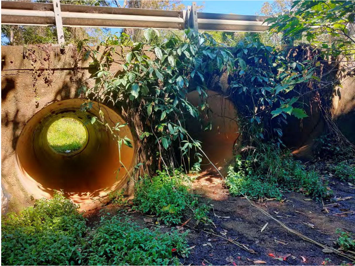
Plate 1 – 3 X 1500mm pipes convey the western tributary of Moogurupum Creek under Double Jump Road
