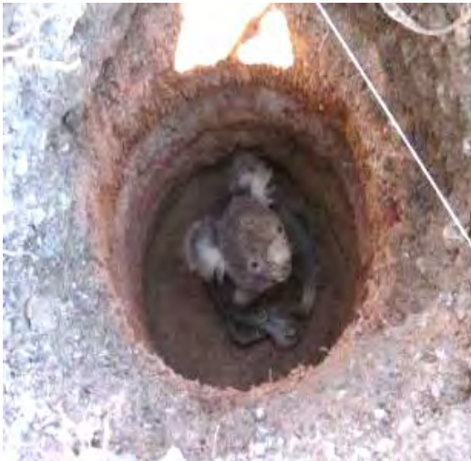
Figure 4.4.8. (photo D de Villiers) Deep post holes for koala proof fencing along a state road upgrade entrapped a koala that could not climb out of the hole.
