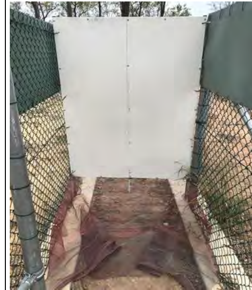
Figure 4.3.18. (photo: Jonathan Hanger) A skirt of netting allows a koala to push underneath the fence but cannot easily be lifted for koalas to travel in the reverse direction.
