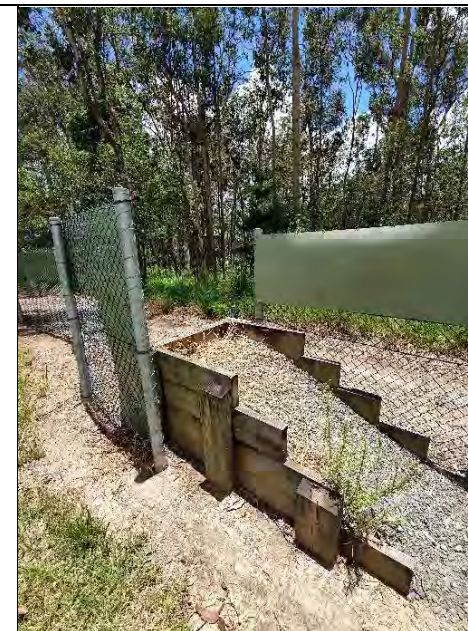
Figure 4.3.23. (photo D de Villiers) A koala escape ramp may assist to funnel koalas into secure bushland.
