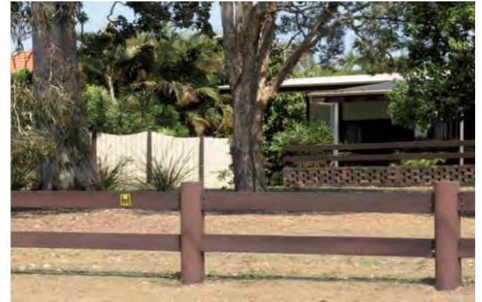
Figure 4.1.1 Post and rail fencing provides the most permeable fencing solution for koalas.
