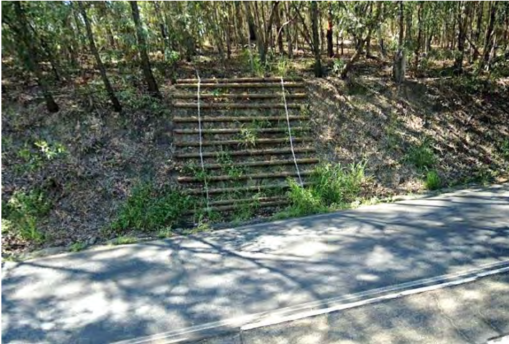
Figure 4.3.24. (photo: google earth). A koala escape ladder is installed on a steep embankment to facilitate rapid egress by koalas from the road corridor in a known koala crossing location.
