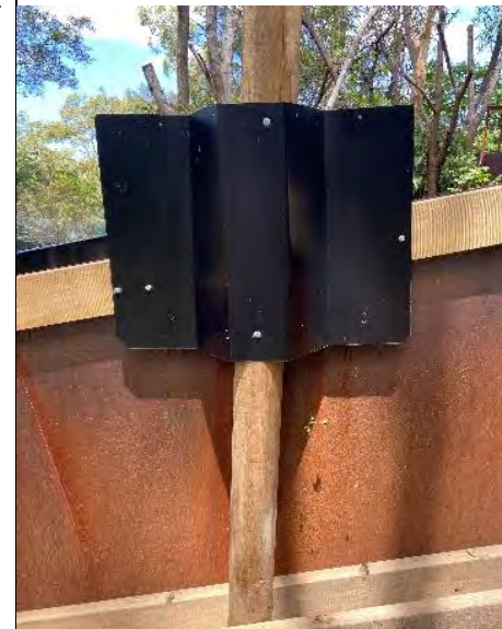
Figure 4.2.4. (photo David Fleay Wildlife Park) Fencing supports fitted with a 'koala shield' prevents koalas climbing the support.
