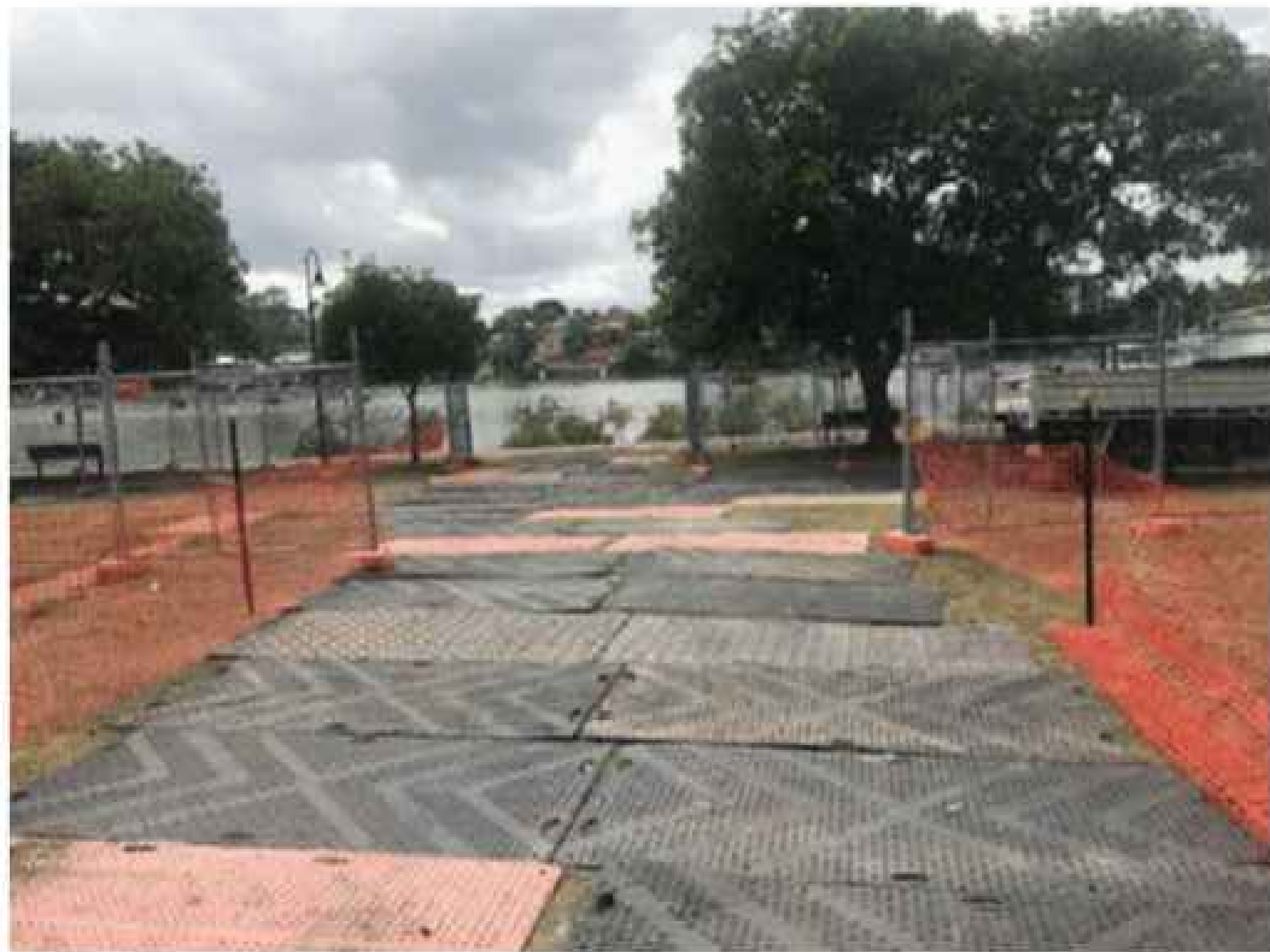
BRIDGING BOARDS OVER TREE PROTECTION ZONE (EXAMPLE)
